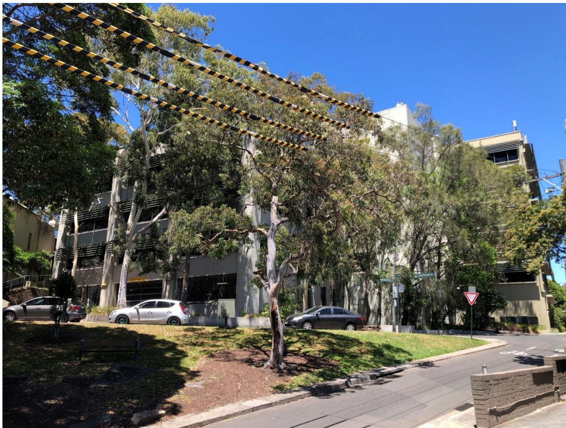
site viewed from Stewart Street
